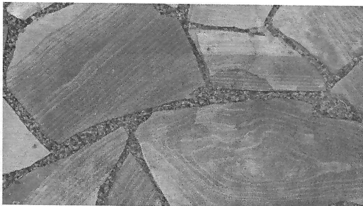
The beautifully striated rose limestone floor for the future arbor has already been laid by mason and neighborhood resident, Bob Howard.
